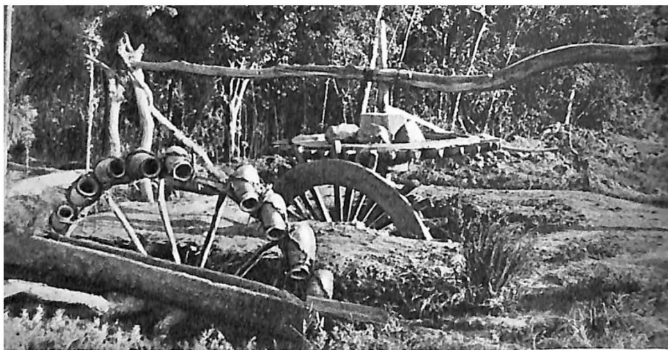
This is a "chigir," an installation which in the old days used to bring water to the fields
