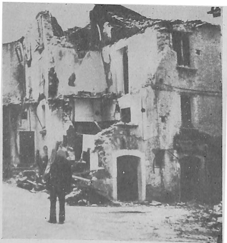
Fig. 7. Damage to buildings due to November 23, 1980 earthquake (magnitude 6.9) in Italy.
