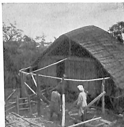
Construction of the frame of the Ka Kyndur
