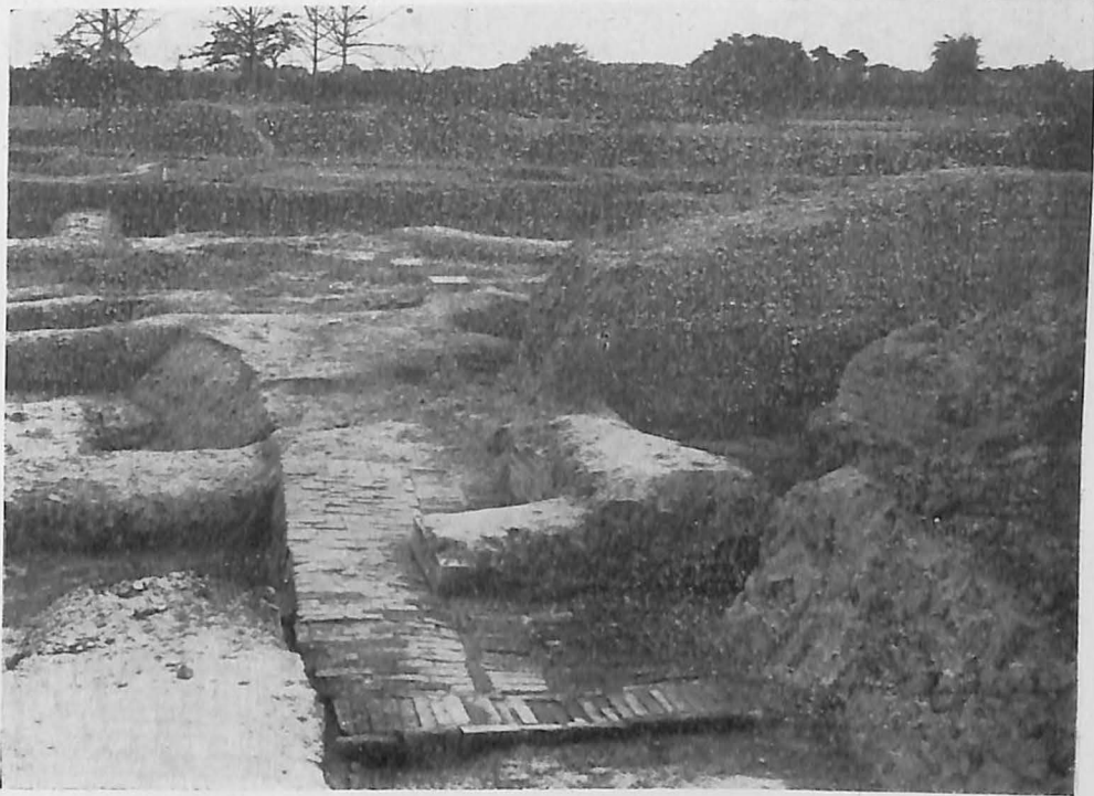
(a) Pavement of brick-on-edge, Str. II, Tr. 5
