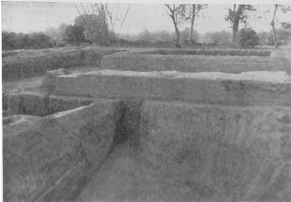
(b) Foundation of a temple (?) built above Structures of Str. III, Tr. 8.
