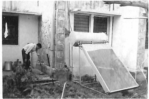
Domestic Solar Water Heating System.
