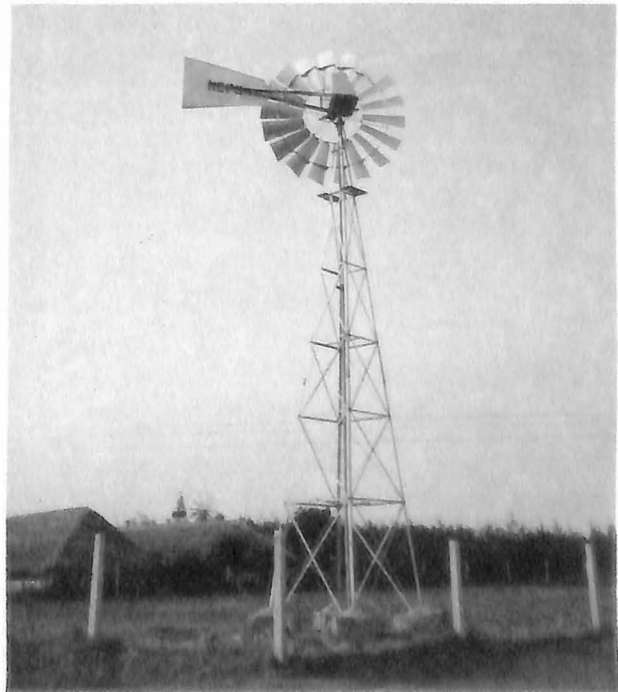
Gear-type Wind-Mill for Water Pumping.
