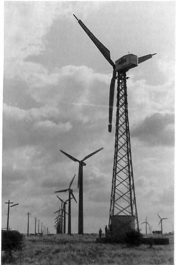
BHEL 200 KW Wind Electric Generator at Kayathar.
