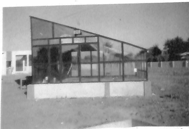
Solar Timber kiln for quality wood seasoning.
