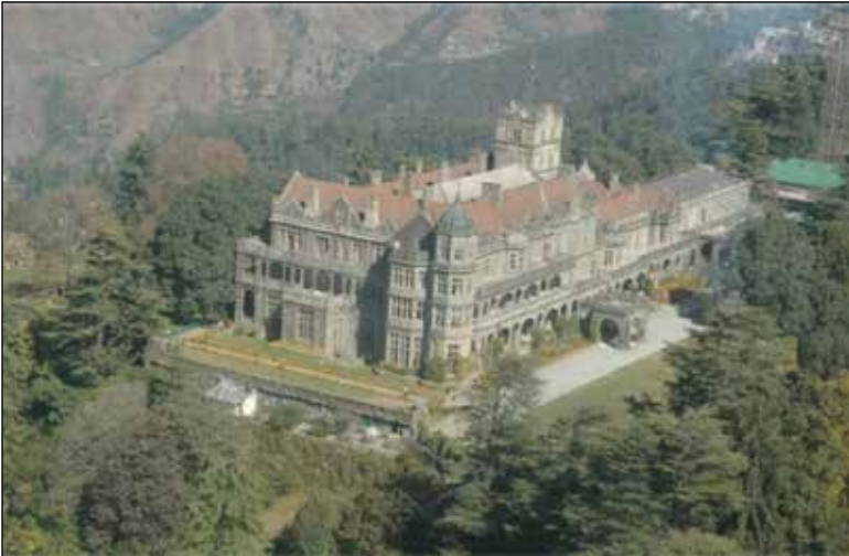
Aerial view of Viceregal Lodge, Shimla
