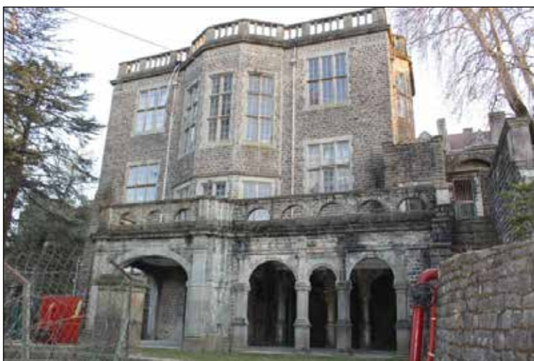
View showing: Council Chamber
