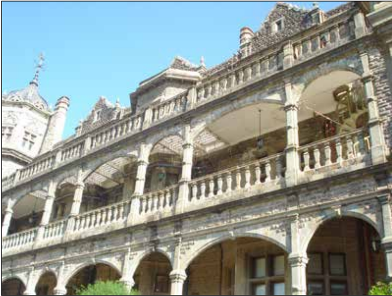
Exterior view from the south showing covered verandas and arcades
