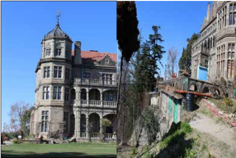
View of south west Tower and Carpenter's workshop at basement level
