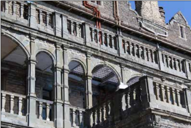
View showing arcade at first floor level above Band porch
