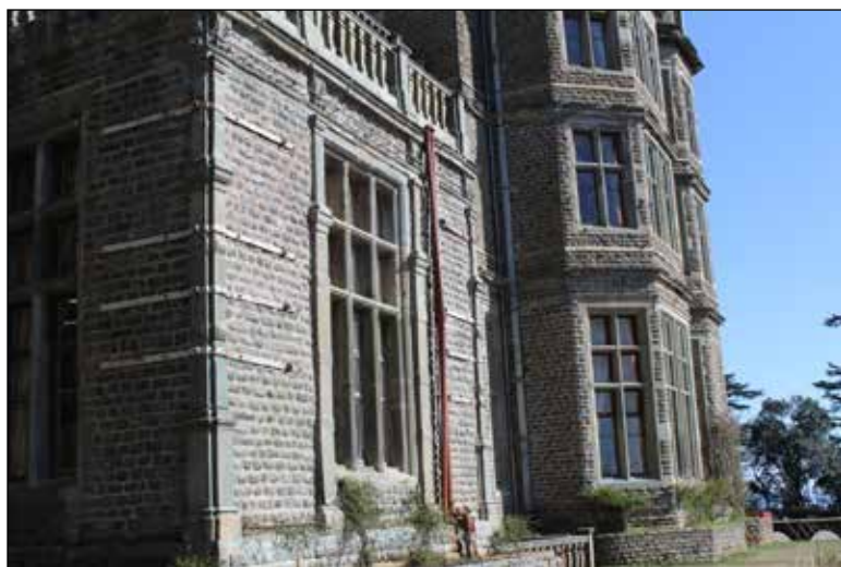
View of west façade and Band porch
