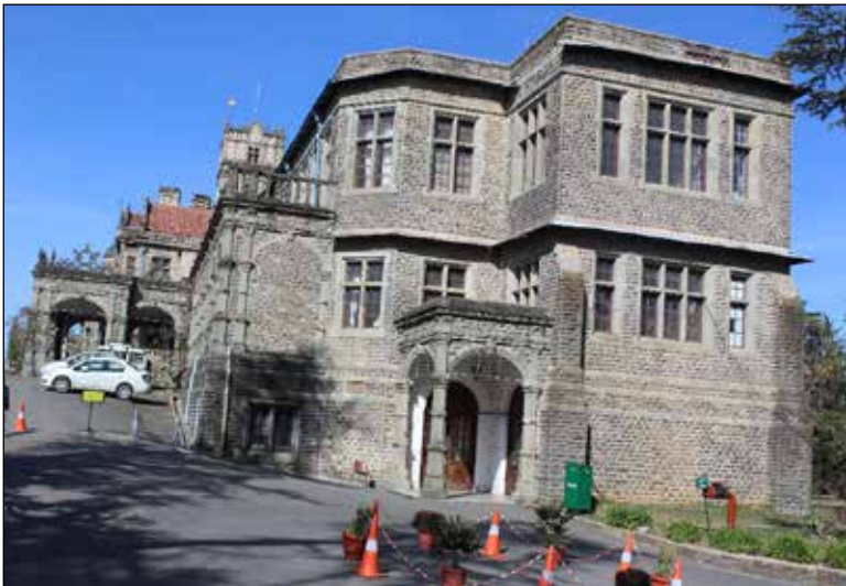
Public Entry Building, view from the east
