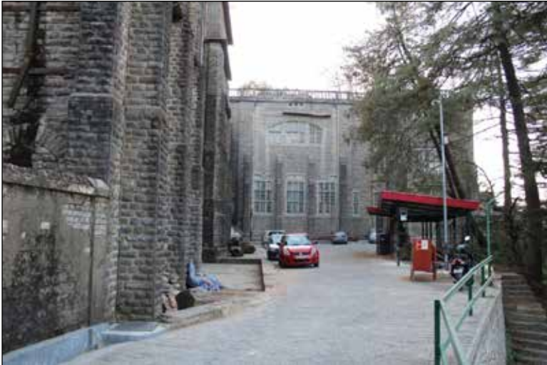
Side view of the Kitchen Wing and Council Chamber
