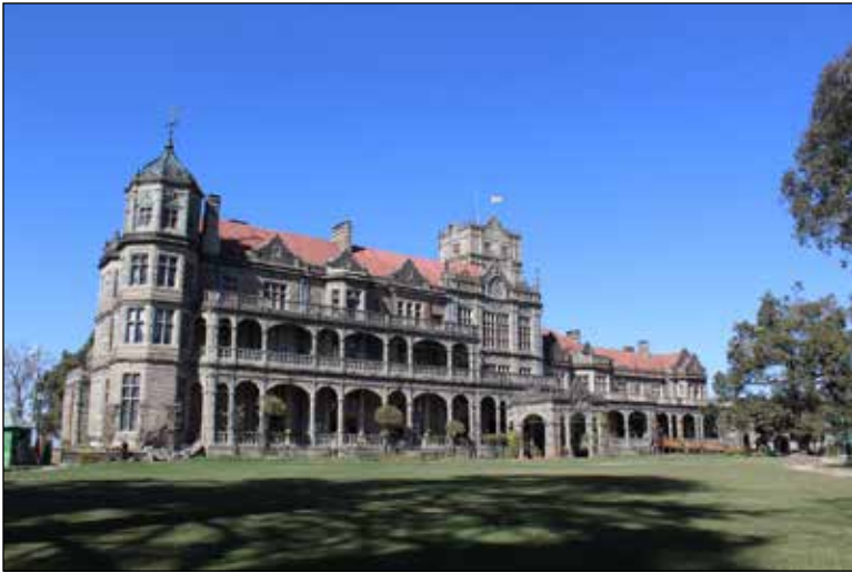
View of the façade on south side
