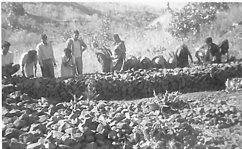
Gabion Structure To Conserve Soil and Water
