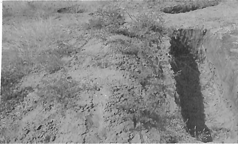
Arresting Water Run Off Through Trenching and Vegetative Measures
