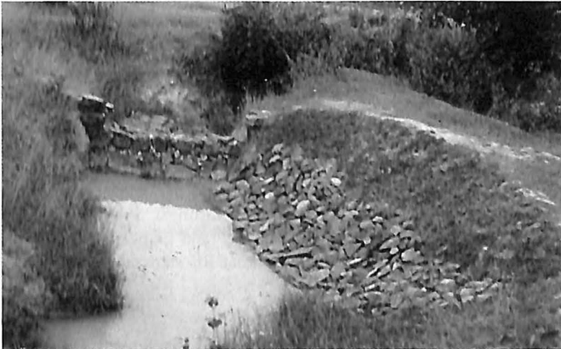
Damming the Stream
