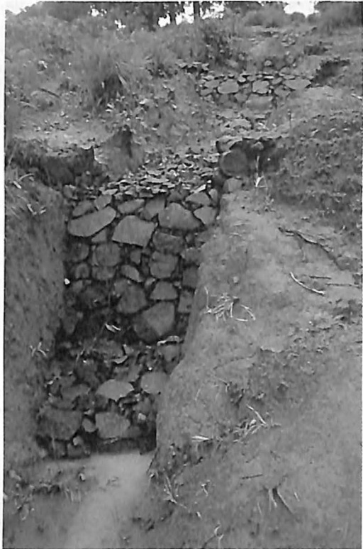
Gully Control Structure
