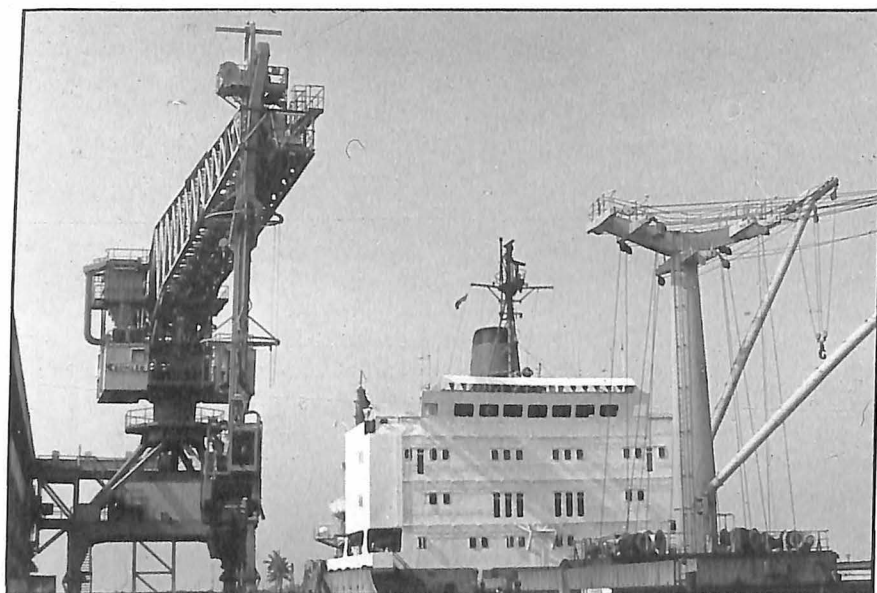
Mechanical ship unloader of Paradeep Phosphates Ltd.
