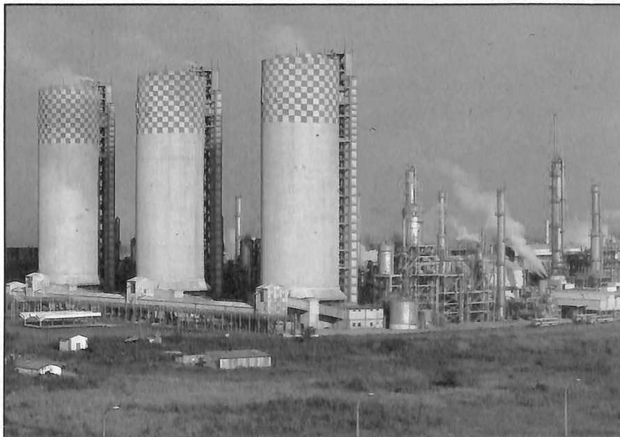
A view of ammonia-urea plant of RCF at Thal (Maharashtra)
