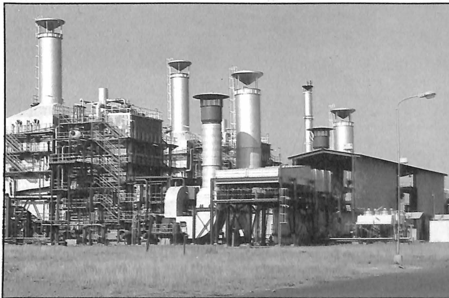
Captive Power Plant of Vijaipur Plant of NFL.
