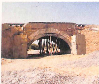
Strengthening of arch bridge for gauge conversion.
