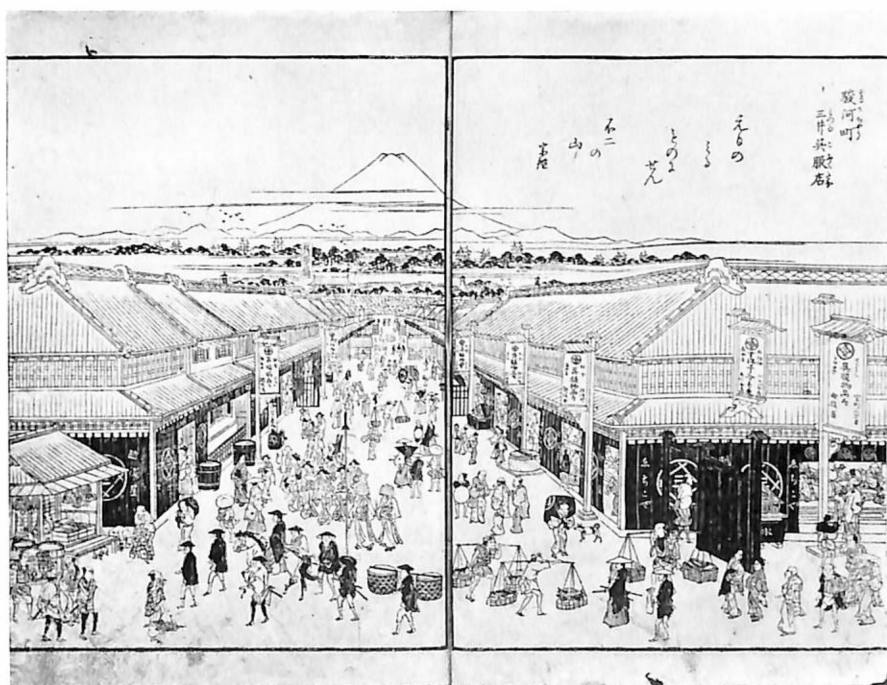
The interior (A) and exterior (B) of the Mitsui dry-goods store at Suruga-chô near Nihombashi in Edo.
