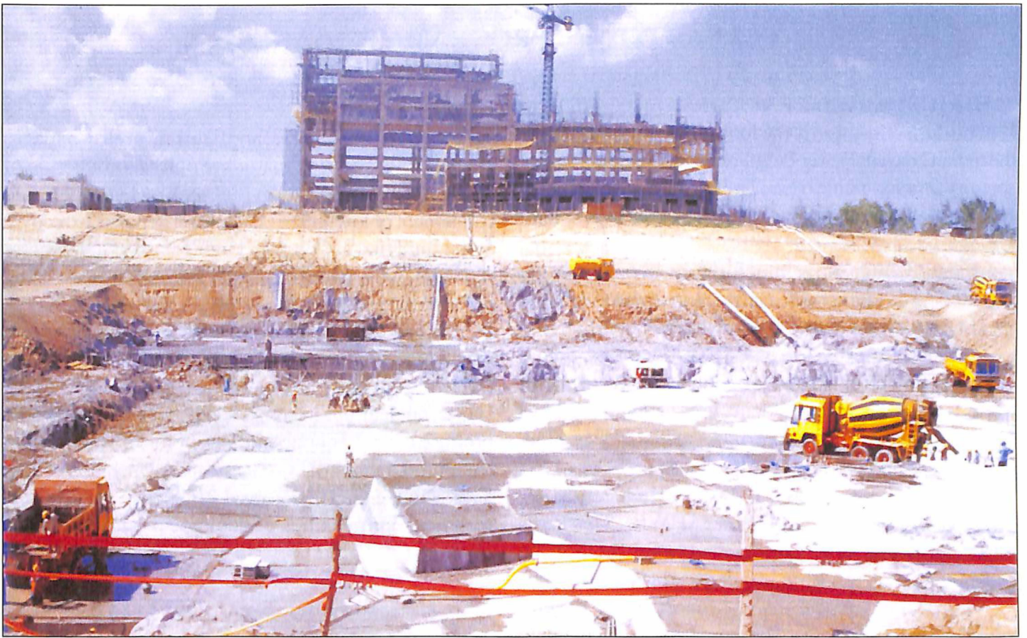
Mud mat filling at Prototype Fast Breeder Reactor excavation
