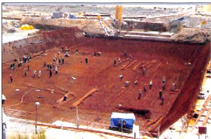
Rebar laying of Reactor Containment Building & Steam Generator Building
