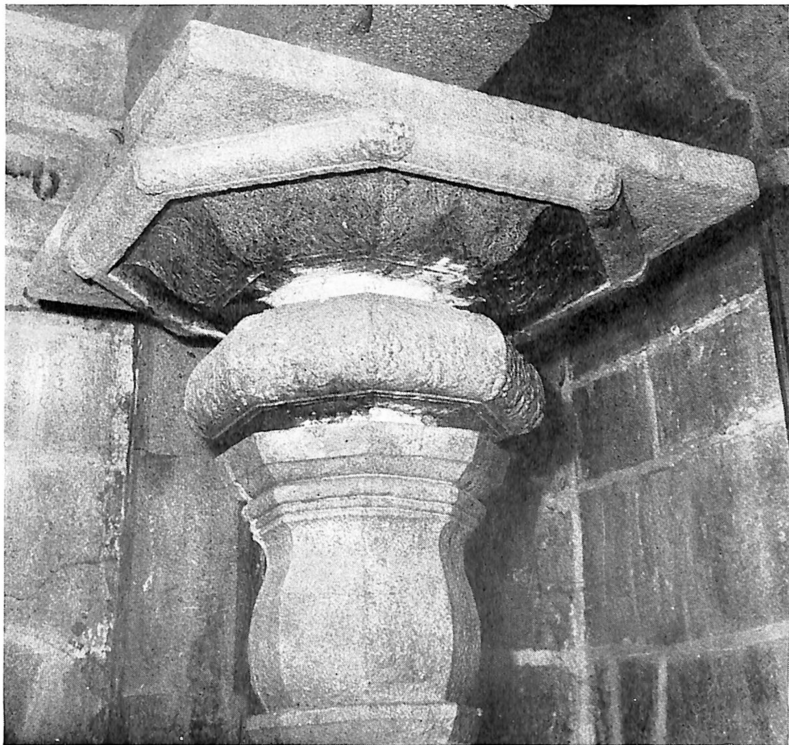
Plate 12 : Kuranganátha. Pillar inside the ardhmandapa. A typical Chola column showing the lower pot-like Kumbham, the Kalasam and the lotus shaped abacus topped by the expanded palagai.
