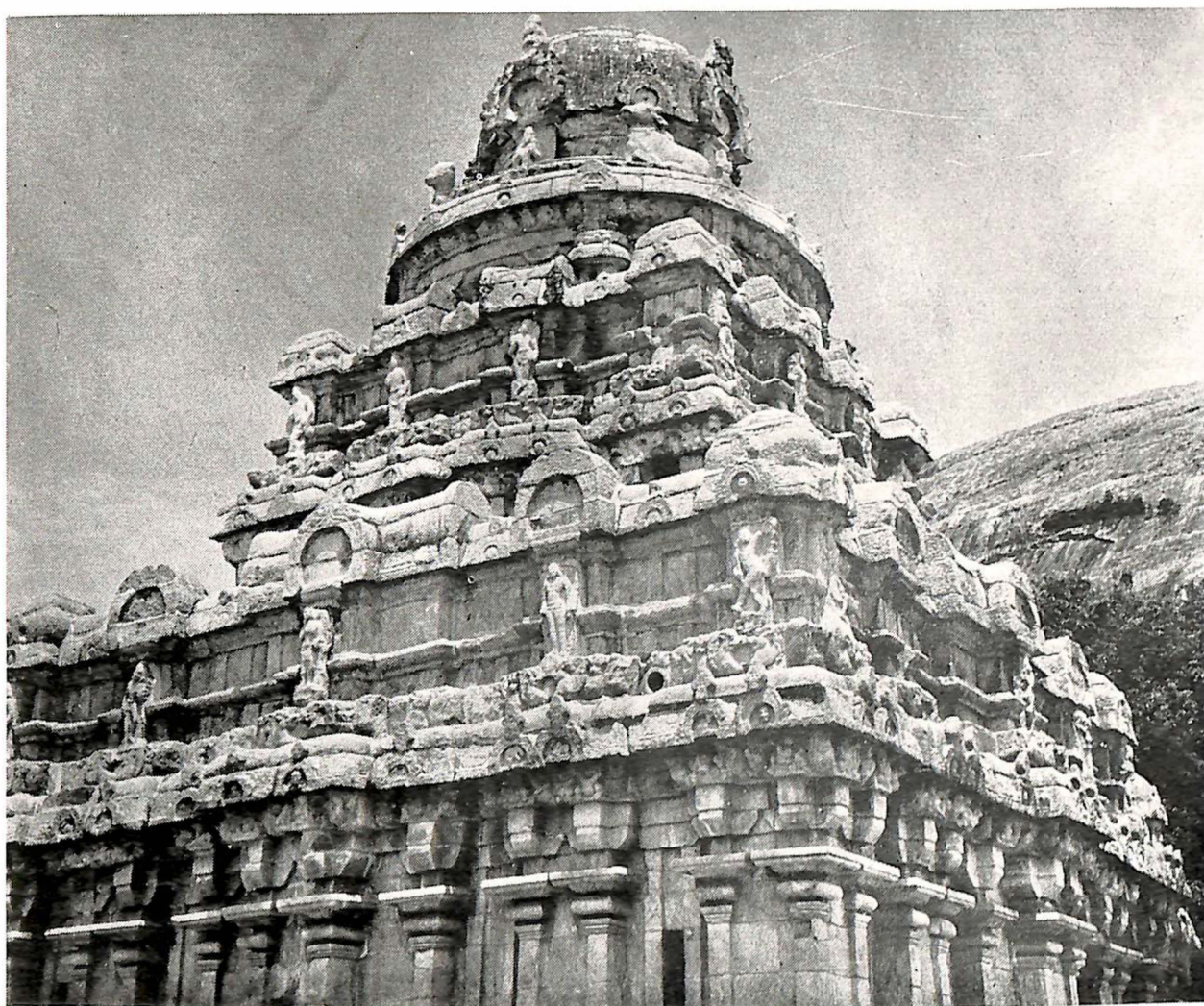
Plate 3 : Vijayālaya Cholisvara. A close view, showing the pilasters, the capital topped by the palagai, angular cut in corbels, the line of ganas under the roll cornice, the little chaitya windows and the goddesses on the parapet walls.
