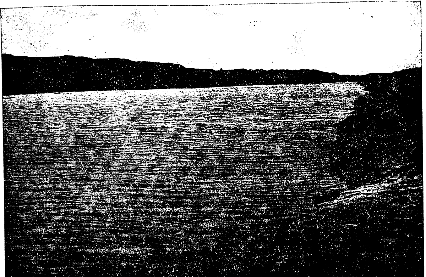
Figure 18. PHOTOGRAPH OF THE NAVIGATION-IRRIGATION CANAL AT DURGAPUR.
