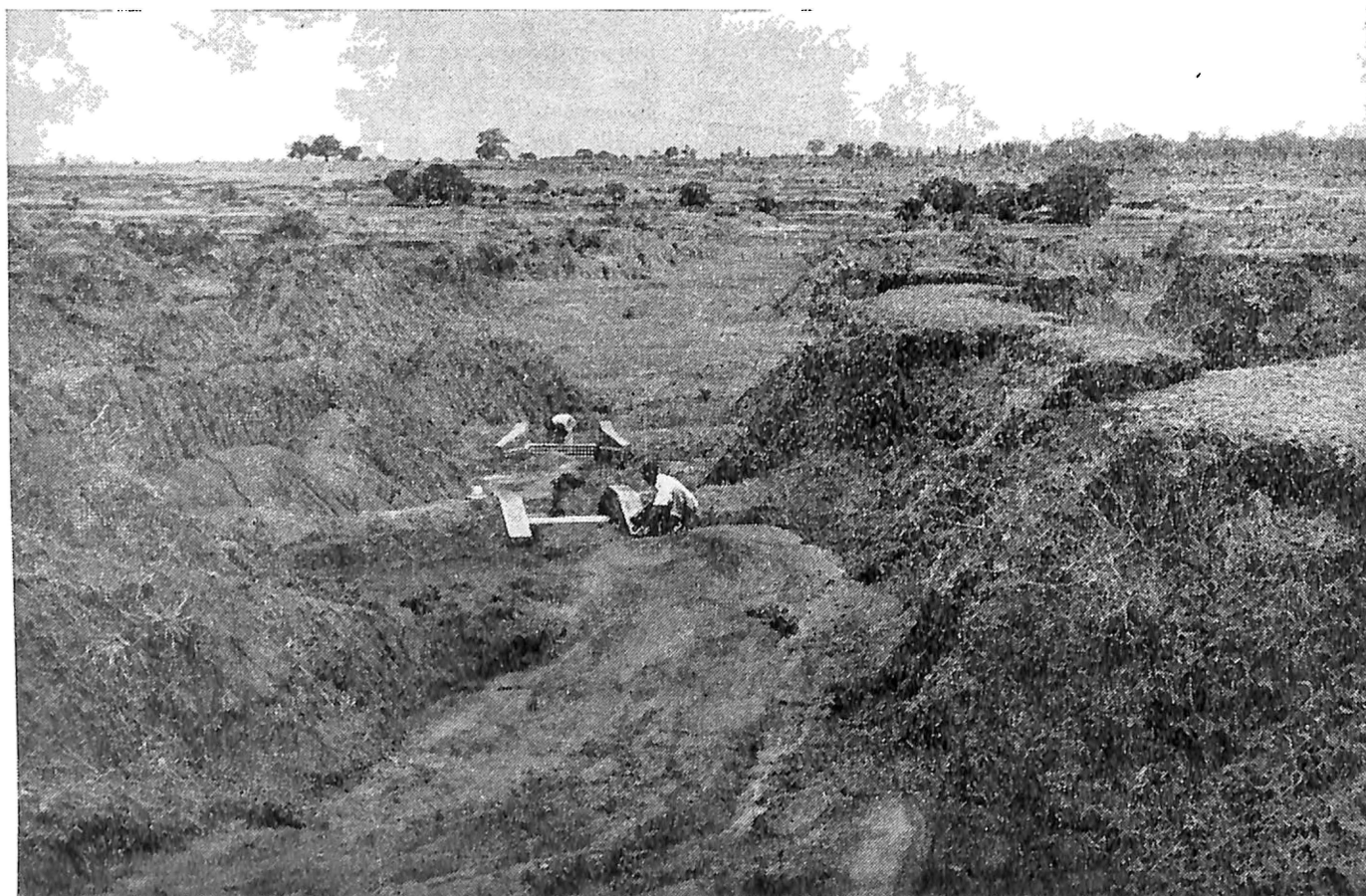
Figure 2. PHOTOGRAPH OF UPPER VALLEY ANTI-EROSION STRUCTURES
