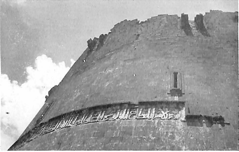
DIYARBEKIR S.W. WALL
