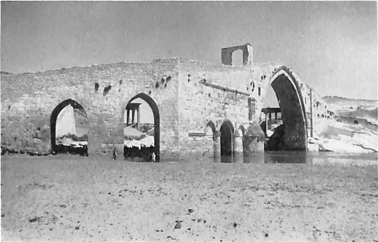
ABASSID BRIDGE E. OF SILVAN ON BATMAN SU: 1147 A.D.
