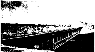
Tilaya dam of D.V.C. : View of the dam from the river side.
